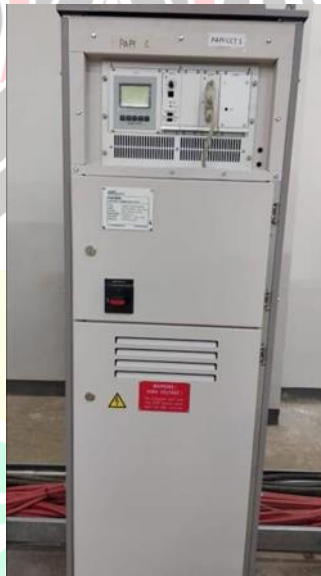
Gambar 2. 1 Constant Current Regulator (Penulis,2021)
